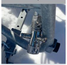
The first-class SnowMaster drain adapters made of stainless steel allow for automatic drainage of the lines when turning off the plant or reducing the pressure to avoid frost damages in the plant and hose lines.
